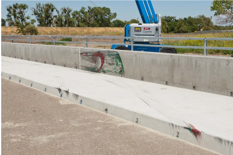
Figure 3-2 – Type 732SW Barrier after Test 130MASH3P13-01
