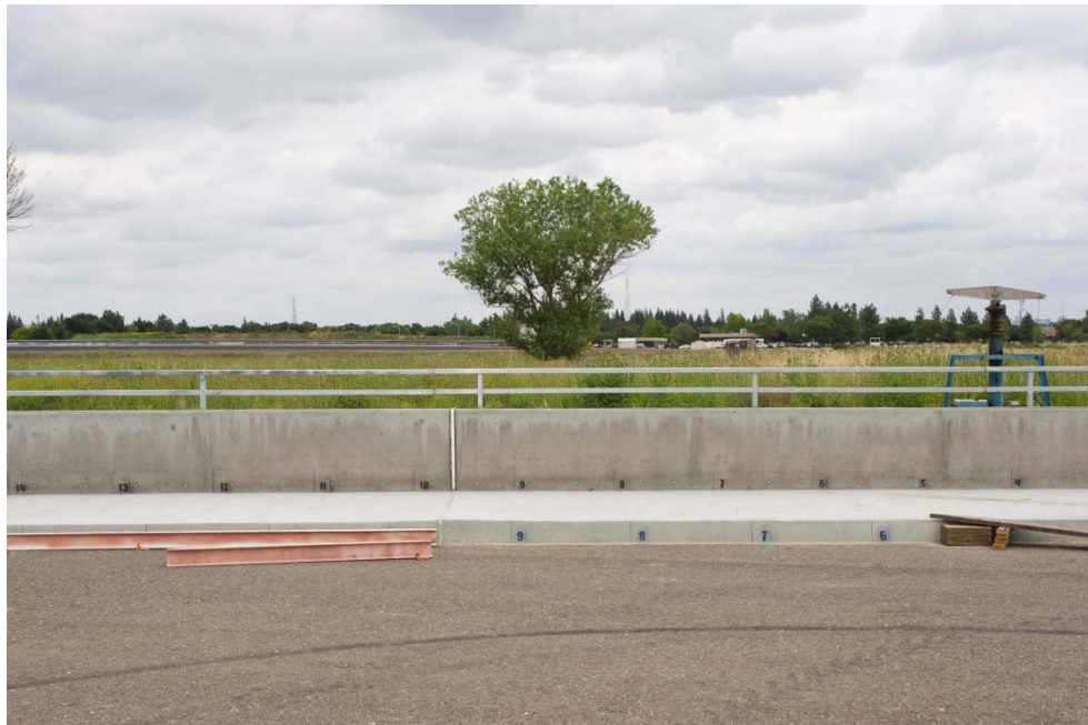
Figure 3-1 – Test article prior to Test 130MASH3P13-01
