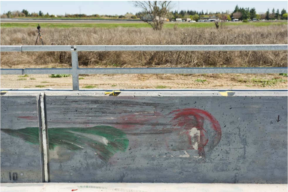
Figure 3-25 – 732SW Barrier face scraping after Test 110MASH2C14-01
