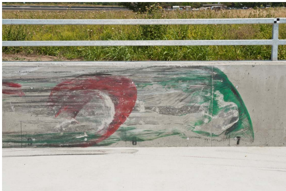
Figure 3-3 – Close-up of 732SW Barrier after Test 130MASH3P13-01
