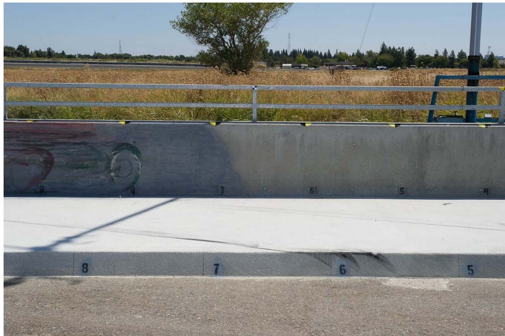
Figure 3-13 – Type 732SW bridge rail face after 130MASH3C13-02
